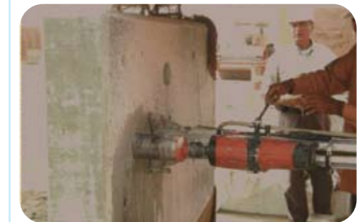
Concrete Core Test
