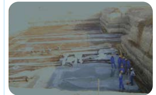
Effluent Storage Tank Blinding
